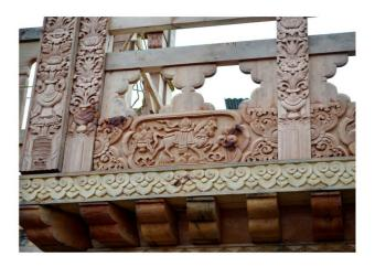
pillars, doors, beams, window frames, and roof girders are fitted separately on the ground. These elements are then joined together using thick wooden pegs. Logs with ledges serve as staircases. Roofs are also made of wooden shingles, weight down in their places by boulders.
